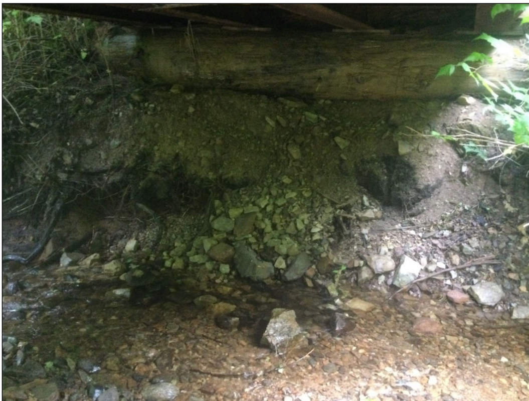
Figure 2.—Eroding river-right bridge abutment at waypoint 2279.
